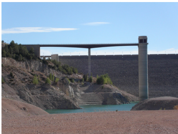
Figure 1.11: Extraction tower and dam of San Clemente Reservoir (Height of tower: ca. 30m).
